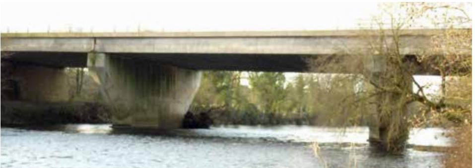
A1M bridge (AB)
