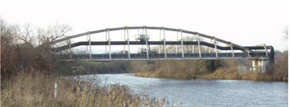
Preston Pipe Bridge (AB)
