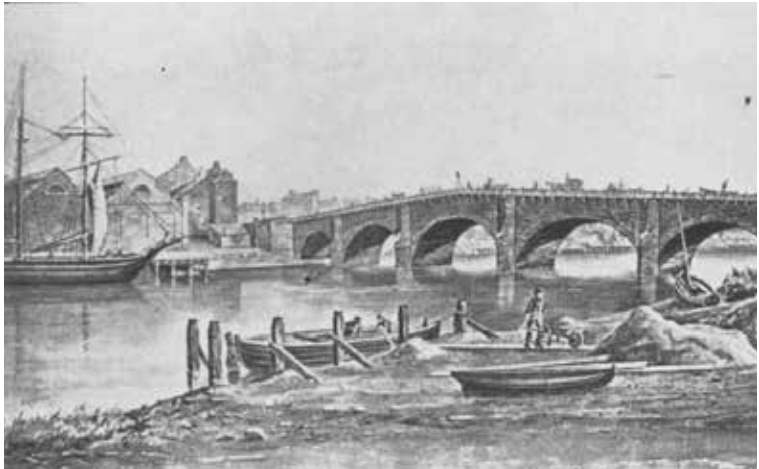
Stockton Stone Bridge (AB)
