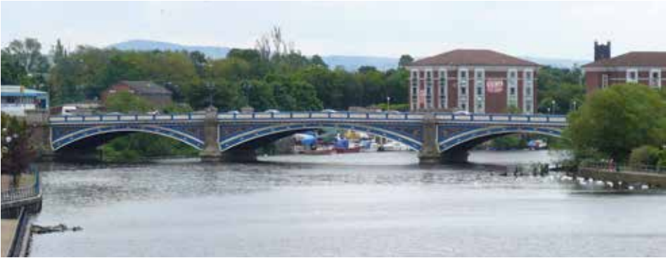
Victoria Bridge (AB)
