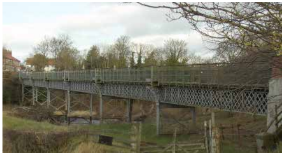
Low Hail Bridge (AB)
