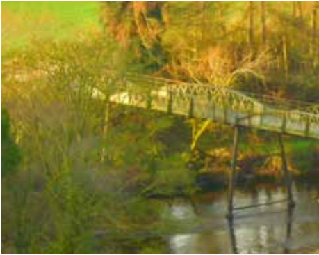
Girsby Bridge (AB)
