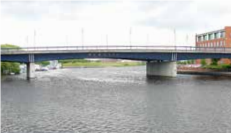
Princess of Wales Bridge (AB)
