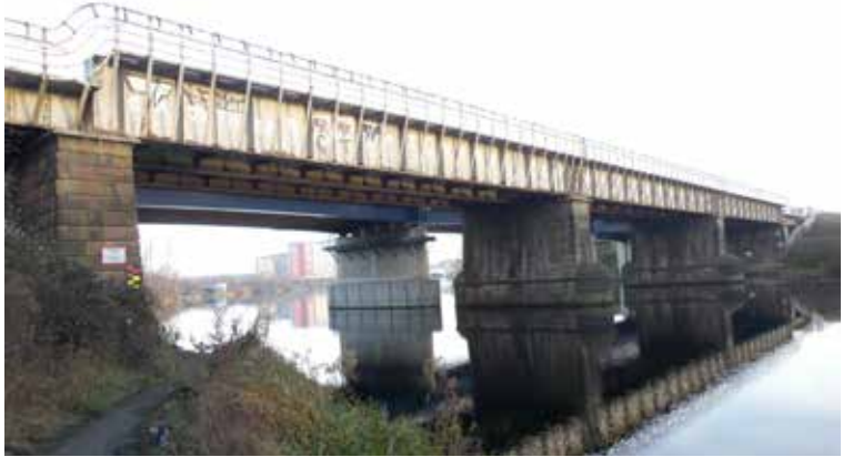
1906 bridge on 1844 stone piers (AB)
