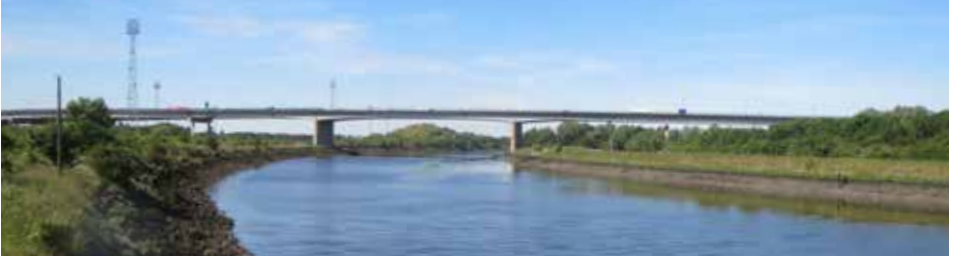
A19 Tees Viaduct (AB)
