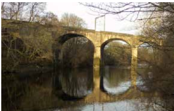
Croft Rail Bridge (AB)
