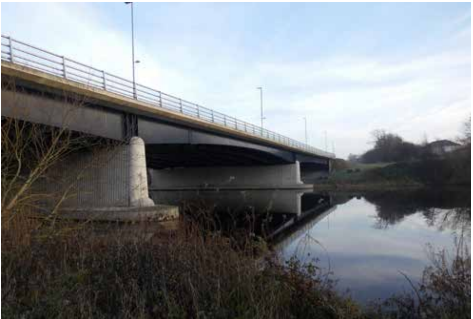
Surtees Bridge (AB)
