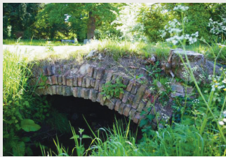
▲ Stainton Beck Footbridge
