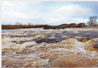
▲ Broken Scar Weir
