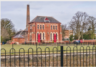
▲ Tees Cottage Pumping Station
