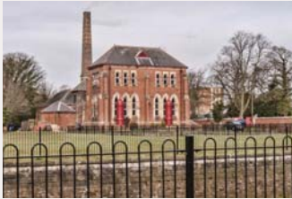
▲ Tees Cottage Pumping Station
