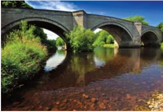
▲ The bridge at Piercebridge
