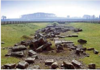
▲ Piercebridge Roman Bridge
