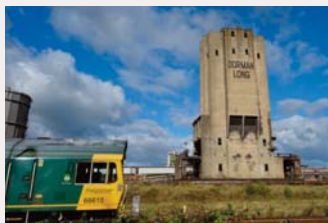
▲ Dorman Long Coal Tower
